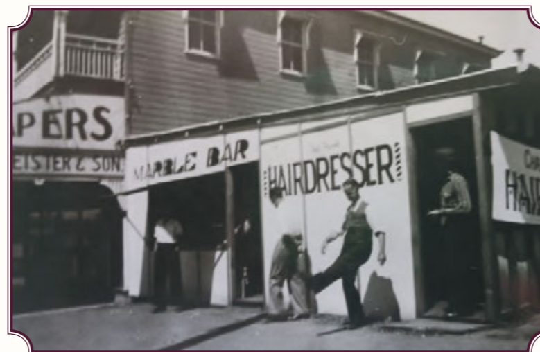
Temporary cafe and barber after fire, January 1940 Photographer unknown
