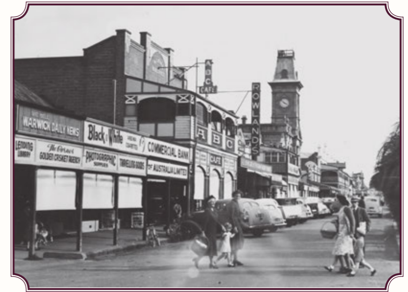
Street scene in Palmerin Street, Warwick, 1949 Photographer unknown
